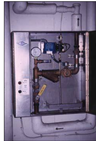
Fig. 2-5 Valve junction panel
