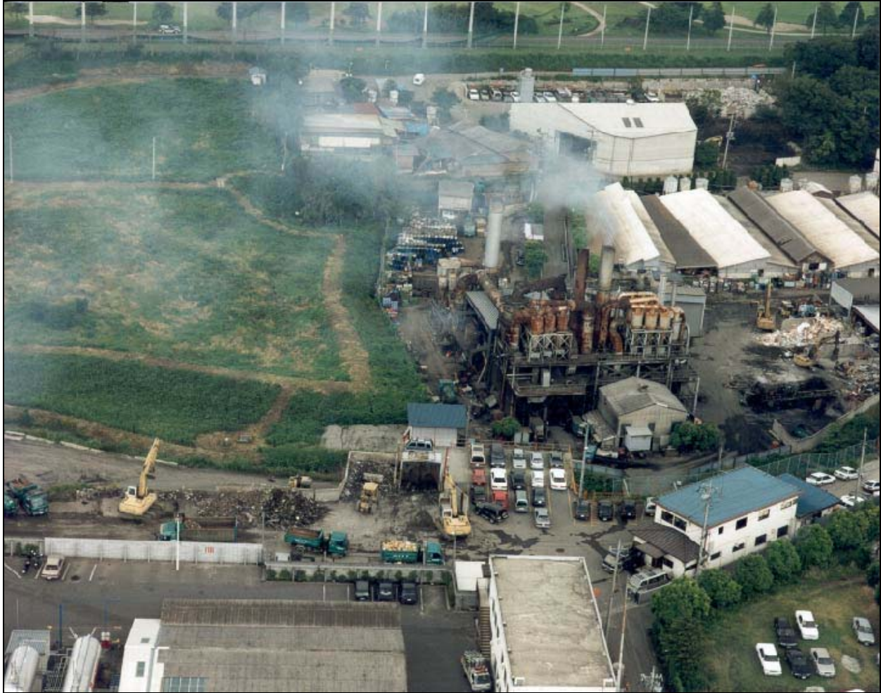
Figure 1-3a — Shinkampo Incineration Complex
